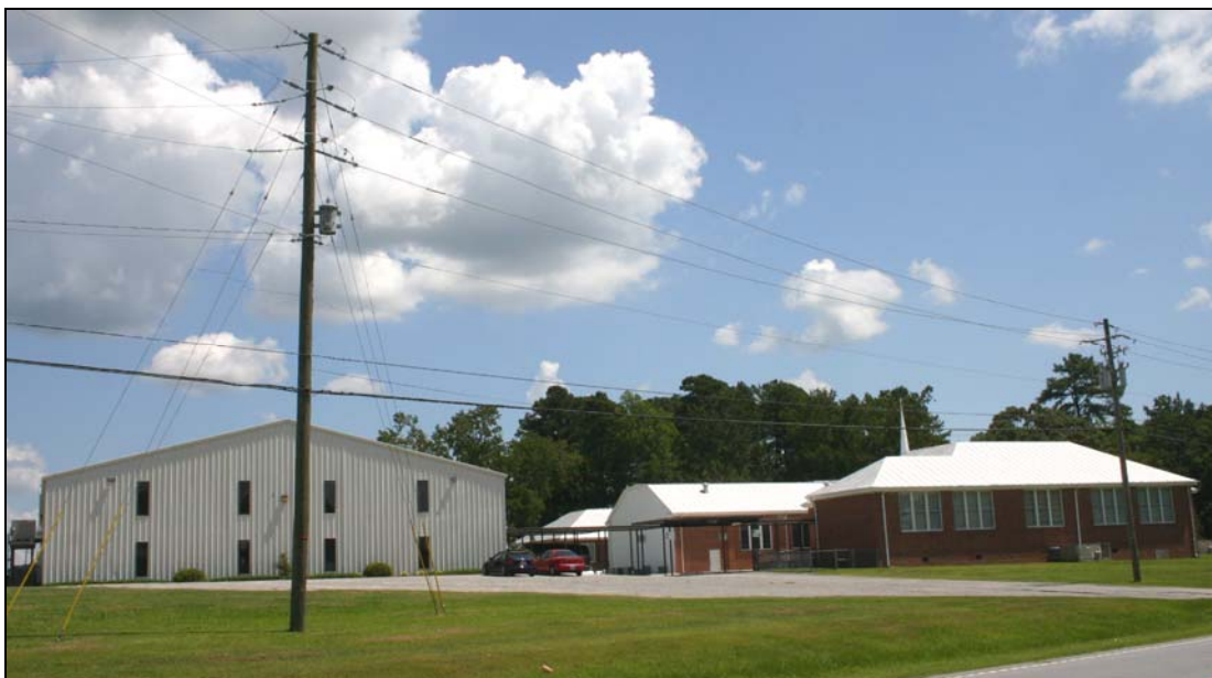
Figure 15: Old Ford Church of Christ, west elevation of former school and overall church complex. Penne Sandbeck, NCDOT, October 2010.
