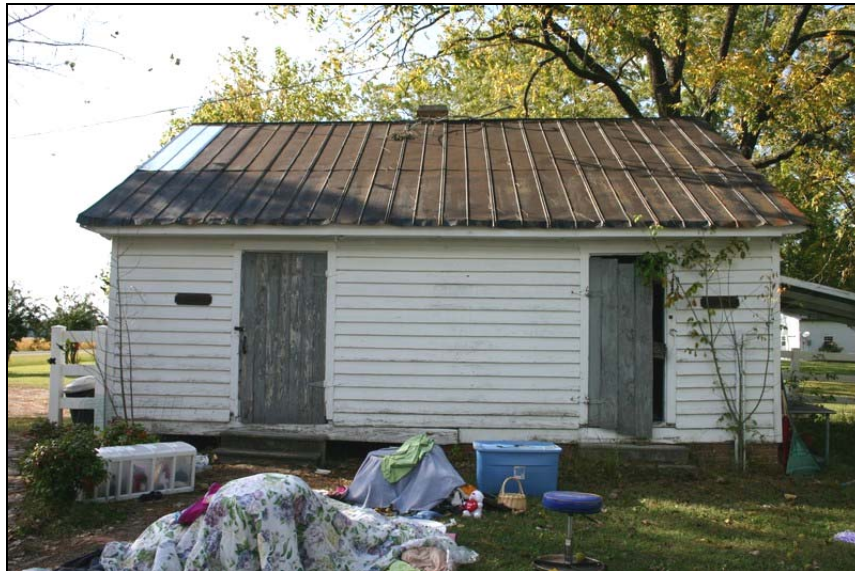
Figure 36: Outbuilding with former washhouse (left) and pump house (right). Penne Sandbeck, NCDOT, October 2010.
