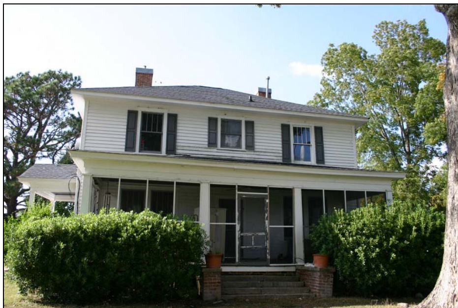
Figure 31: Front elevation of Thad Hodges House. Penne Sandbeck, NCDOT, October 2010.
