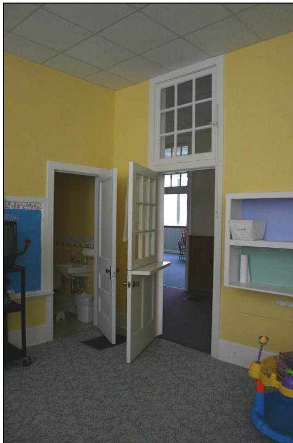
Figure 21: Classroom, showing bathroom, intact dutch door, and transom, Old Ford School. Penne Sandbeck, NCDOT, October 2010.
