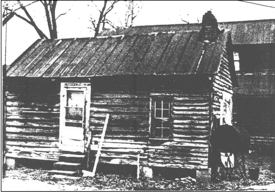
Figure 126: Hadley House, east elevation of kitchen building. Clifton Ellis for NCDOT, 2000.
