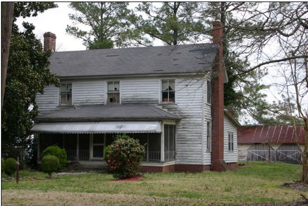
Figure 65: Hodges Homeplace, west façade. Penne Sandbeck, NCDOT, August 2010.
