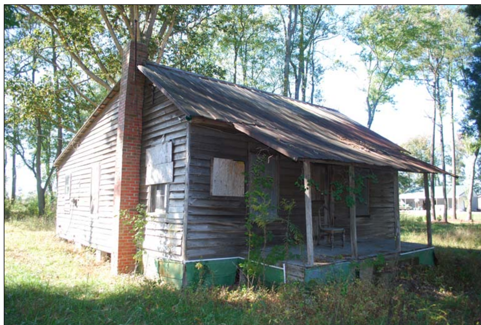
Figure 88: Tenant house (Prop. No. 46), east façade and south elevation. Katherine Husband, NCDOT, October 2010.
