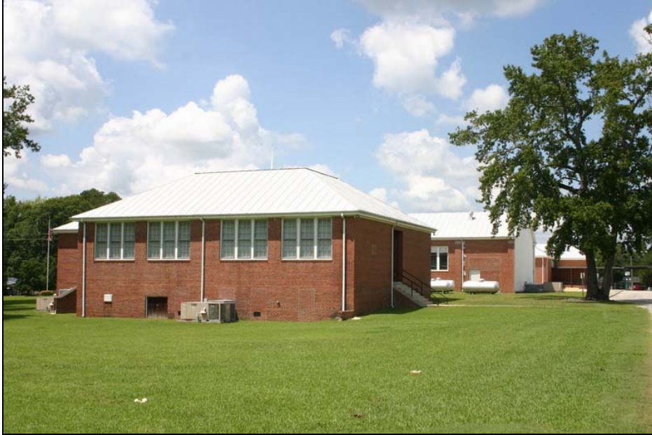
Figure 13: Former Old Ford School, East Wing, east elevation (upperclassmen in this section). Penne Sandbeck, NCDOT, August 2010.
