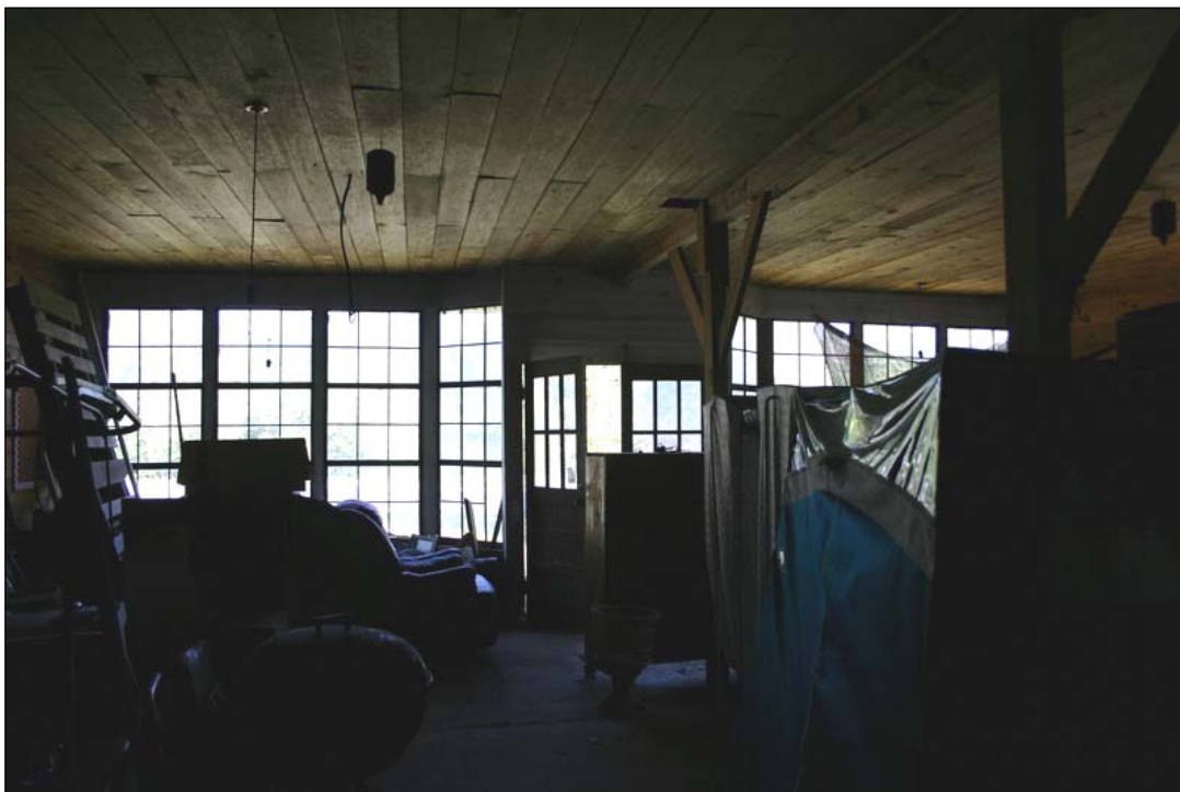
Figure 84: Griffin's Hatchery, interior looking east. Penne Sandbeck, NCDOT, October 2010.
