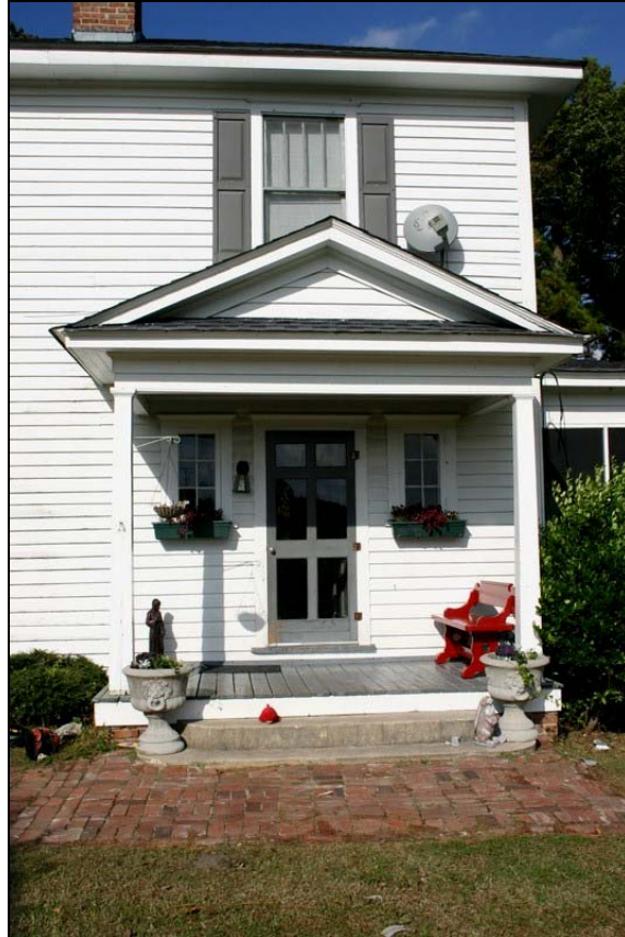
Figure 35: South entrance, Thad Hodges House. Penne Sandbeck, NCDOT, October 2010.
