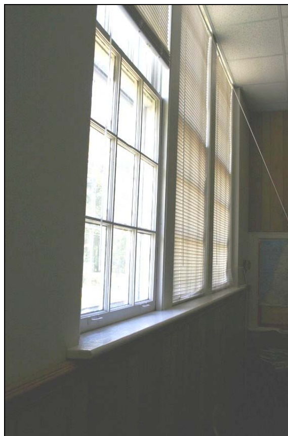
Figure 24: Windows at front elevation are intact. Penne Sandbeck, NCDOT, October 2010.
