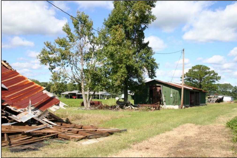
Figure 71: Shed with tobacco barn in foreground, looking north. Penne Sandbeck, NCDOT, August 2010.
