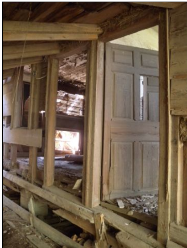
Figure 61: Edwin Gorham House, six-panel door and framing, lathing, and plastering (note that some framing is from when house converted to outbuilding). Brandon McCuin, Gray and Pape, February 2010.
