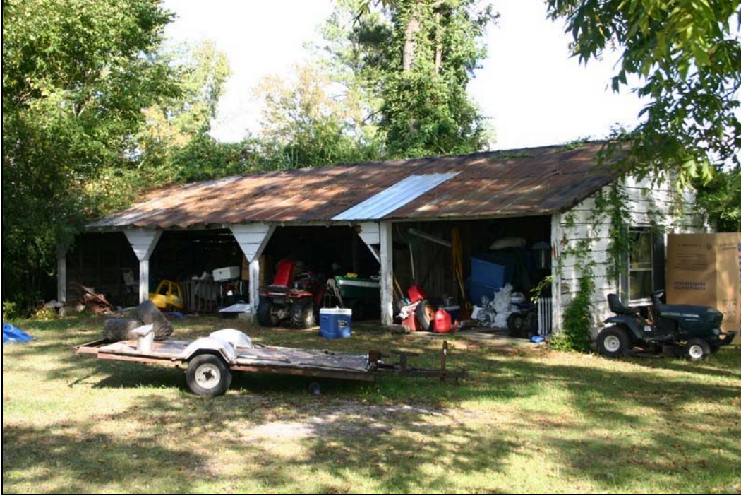
Figure 45: Former equipment shed, Thad Hodges House. Penne Sandbeck, NCDOT, October 2010.
