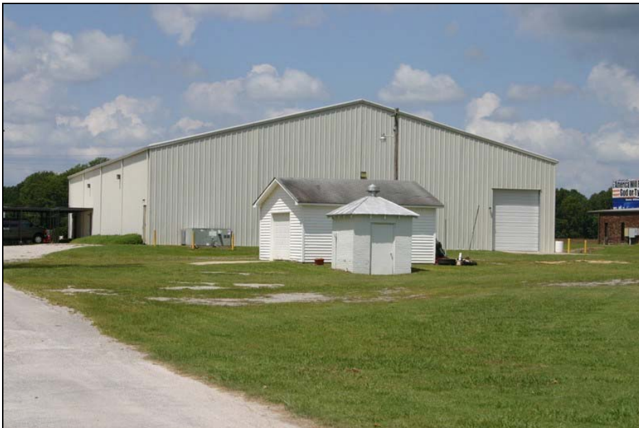
Figure 14: Old Ford Church of Christ, Life Center Building (metal building in background), 1980s shed, and former Old Ford School Pump Building. Penne Sandbeck, NCDOT, August 2010.
