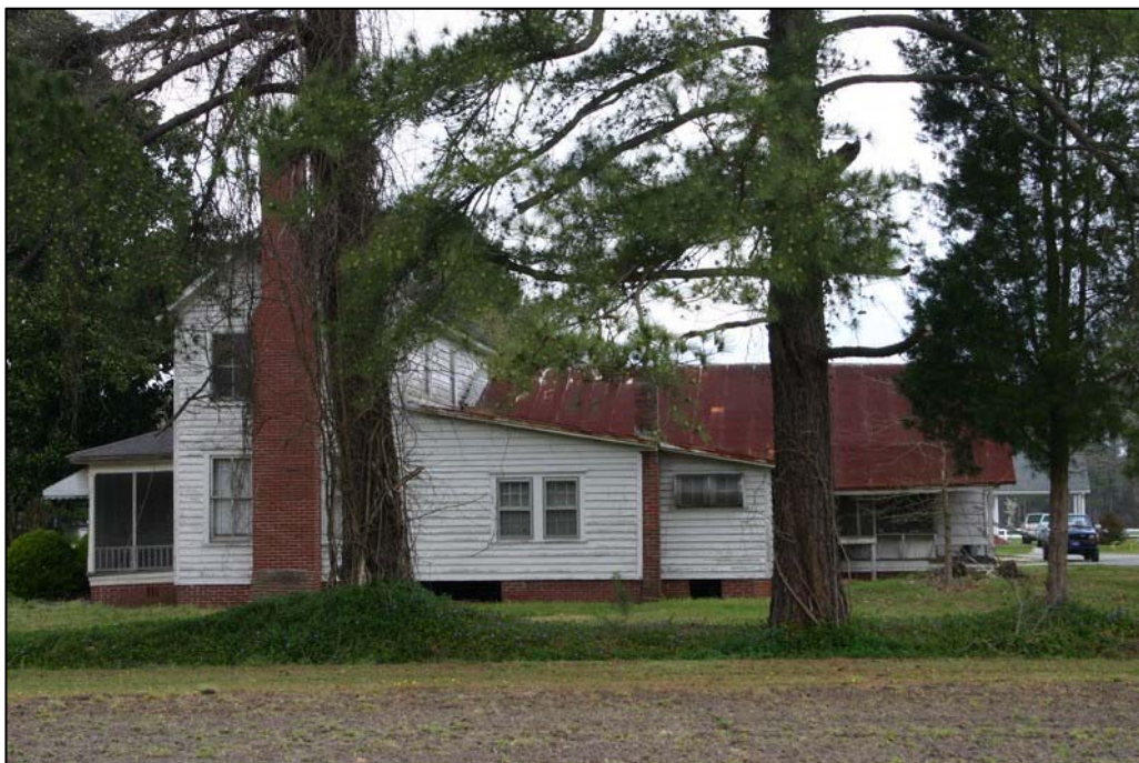
Figure 66: Hodges Homeplace, south elevation. Penne Sandbeck, NCDOT, August 2010.
