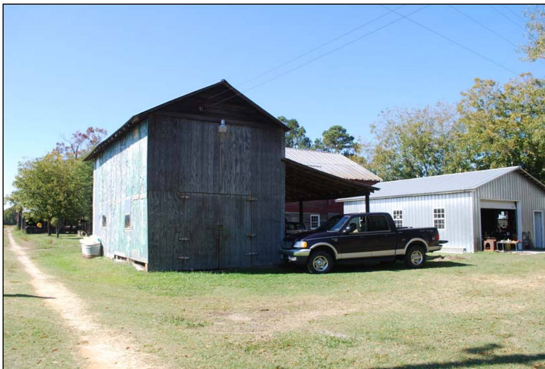
Figure 90: Packhouse and shed on property. Penne Sandbeck, NCDOT, October 2010.
