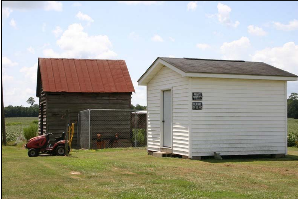
Figure 145: Woolard Perry House, smokehouse and washhouse. Penne Sandbeck, NCDOT, August 2010.
