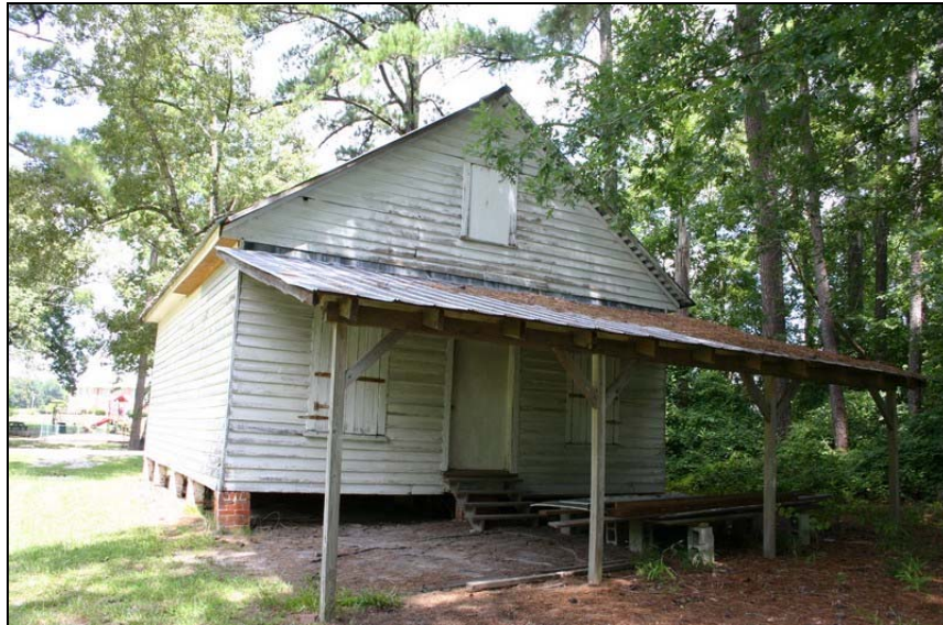
Figure 7: East elevation, Woodmen of the World Lodge. Penne Sandbeck, NCDOT, August 2010.
