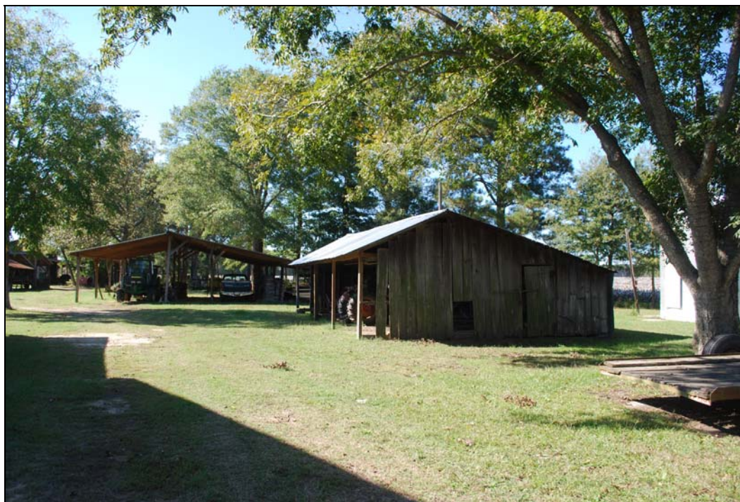
Figure 92: Equipment sheds. Penne Sandbeck, NCDOT, October 2010.
