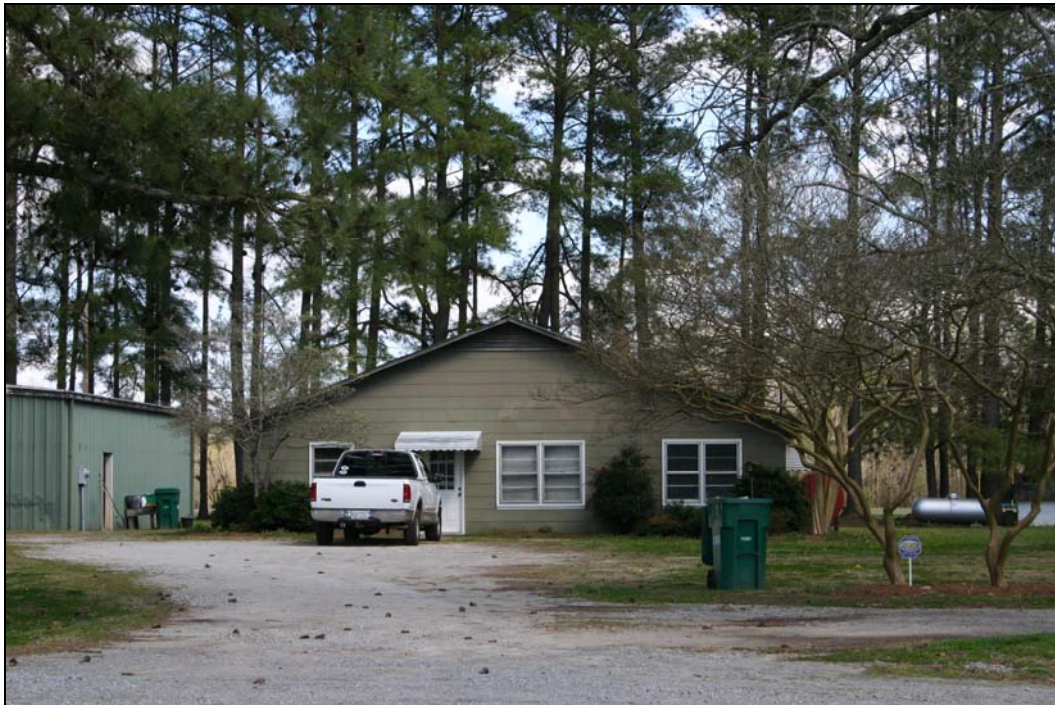
Figure 107: 8111 US 17, west façade. Penne Sandbeck, NCDOT, March 2010.
