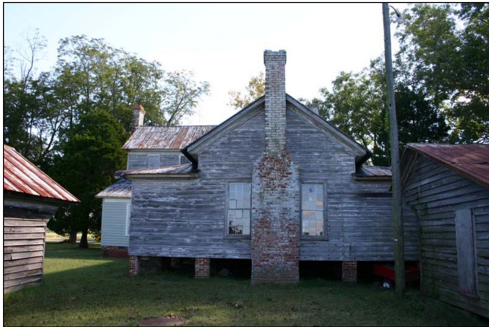
Figure 132: Smithwick-Green-Clark House, west elevation. Penne Sandbeck, NCDOT, October 2010.
