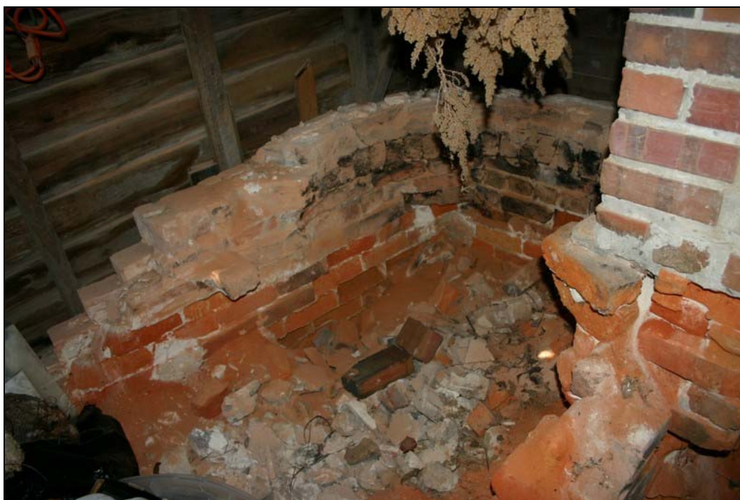
Figure 38: Detail of former washpit for washhouse. Penne Sandbeck, NCDOT, October 2010.
