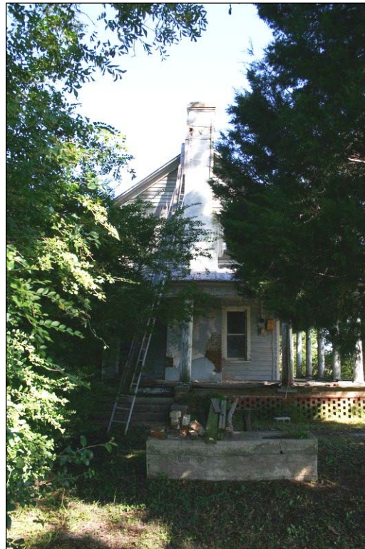
Figure 134: Smithwick-Green-Clark House, south elevation. Penne Sandbeck, NCDOT, October 2010.
