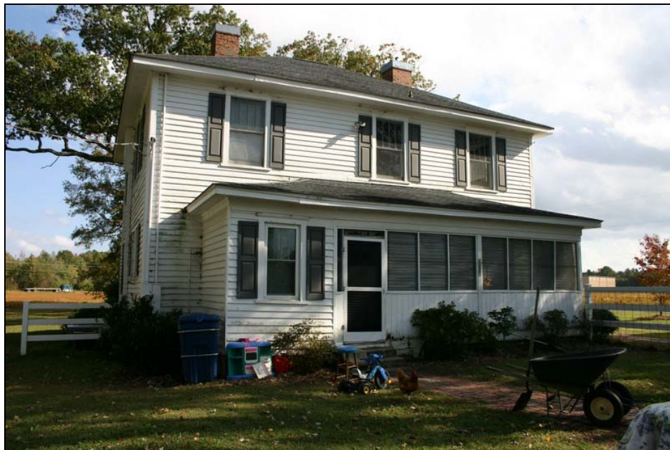
Figure 33: West elevation, Thad Hodges House. Penne Sandbeck, NCDOT, October 2010.
