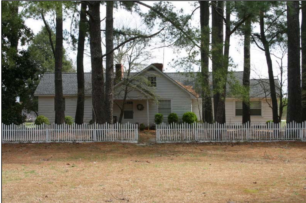
Figure 67: Oscar C. Hodges House, west façade. Penne Sandbeck, NCDOT, August 2010.
