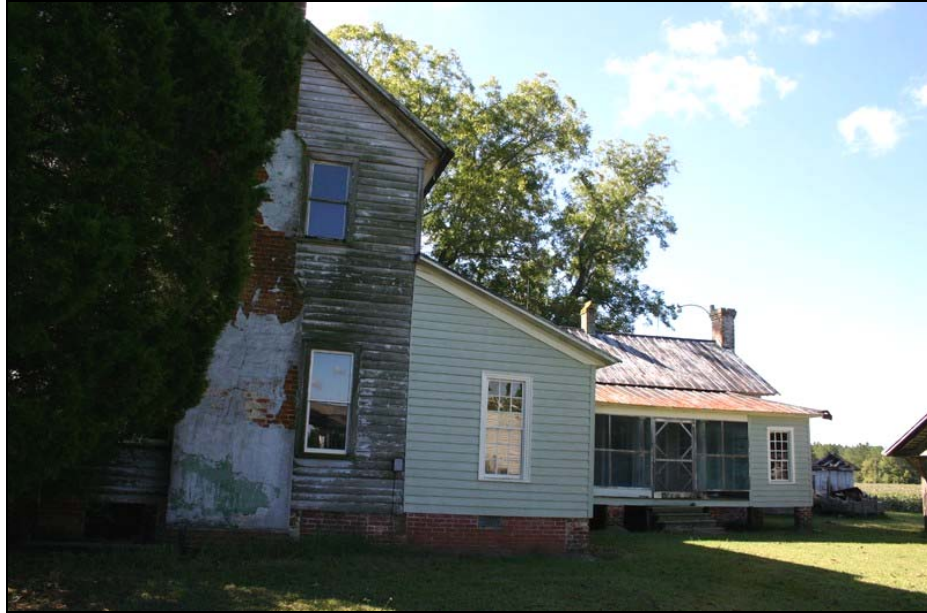
Figure 129: Smithwick-Green-Clark House, north elevation. Penne Sandbeck, NCDOT, October 2010.
