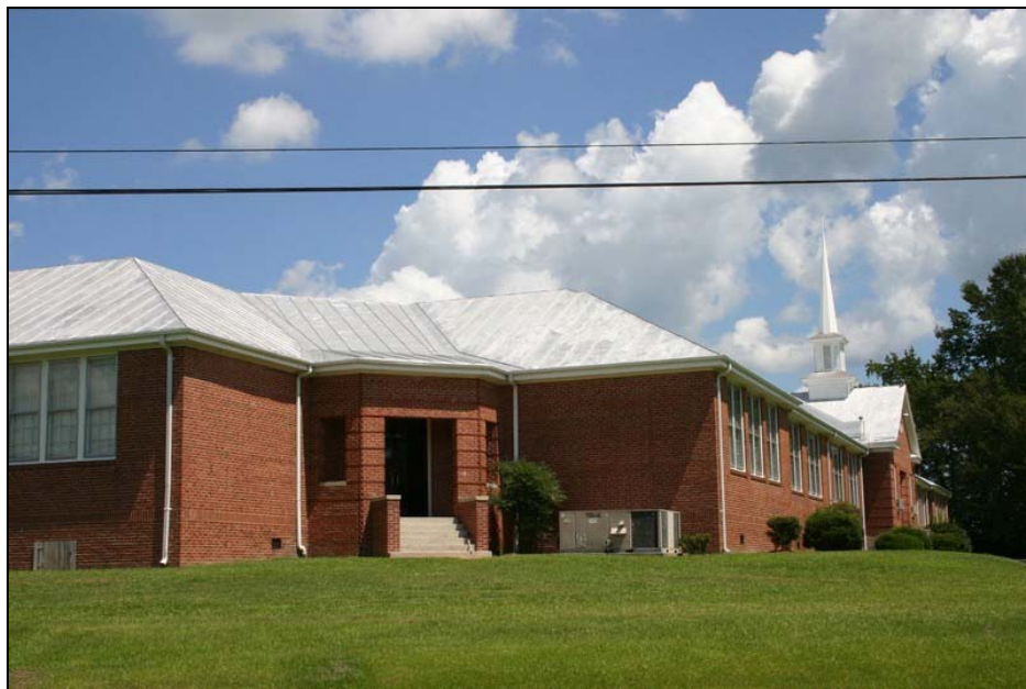
Figure 12: Former Old Ford School, west entrance. Penne Sandbeck, NCDOT, August 2010.
