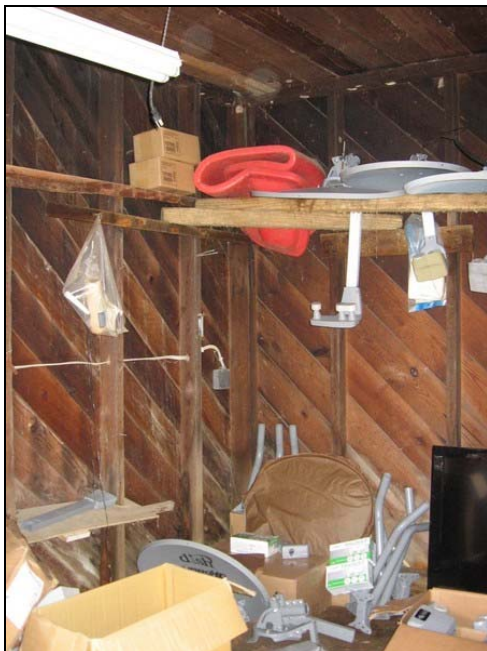
Figure 43: Diagonal sheathing and framing, smokehouse. Penne Sandbeck, NCDOT, October 2010.
