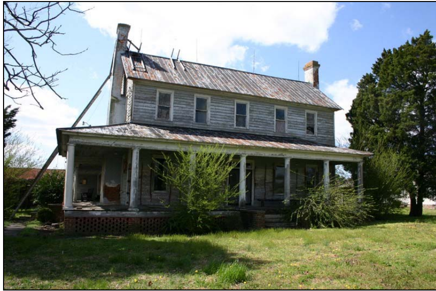
Figure 127: Smithwick-Green-Clark House, east façade. Penne Sandbeck, NCDOT, March 2010.
