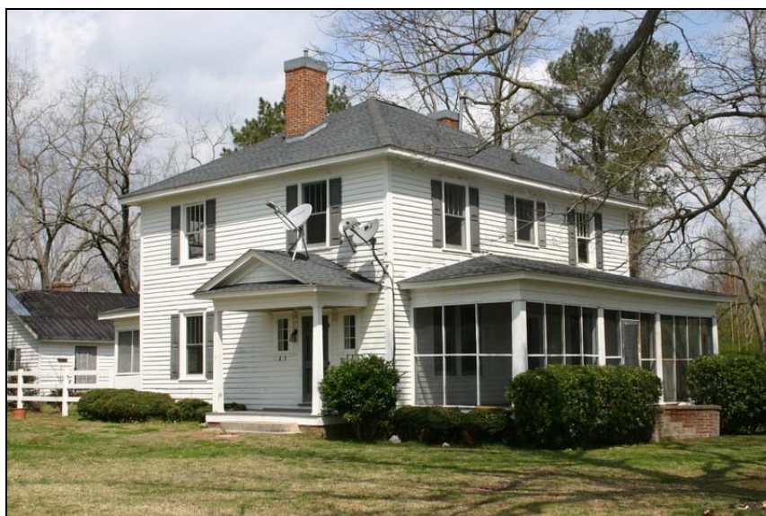
Figure 29: Thad Hodges House, North Side SR 1410, Washington vicinity. Penne Sandbeck, NCDOT, March 2010.
