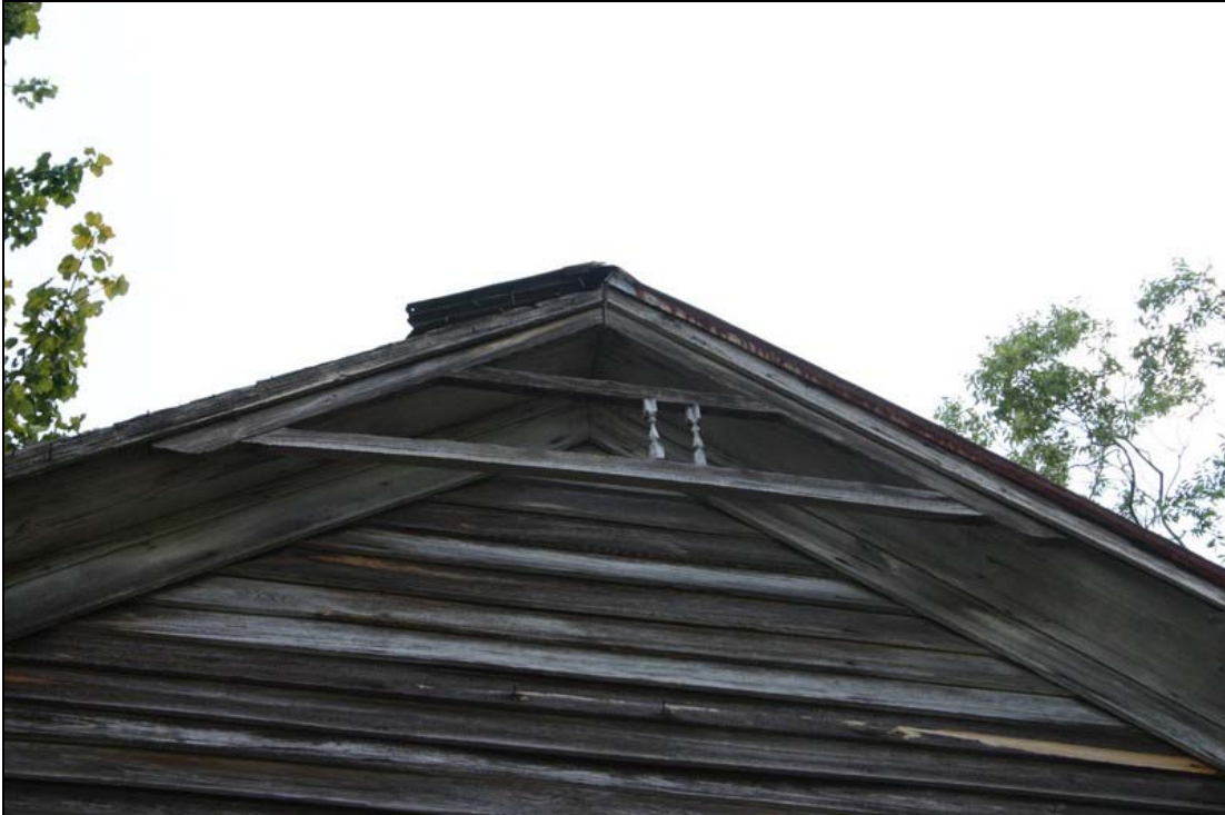
Figure 112: Holliday Store, bargeboard in gable. Penne Sandbeck, NCDOT, August 2010.
