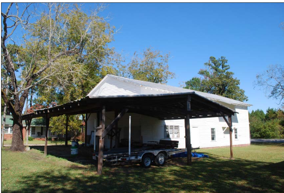
Figure 82: Griffin's Hatchery, west and south elevations. Penne Sandbeck, NCDOT, October 2010.
