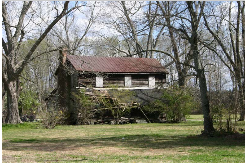
Figure 118: Hadley House, west façade. Penne Sandbeck, NCDOT, March 2010.
