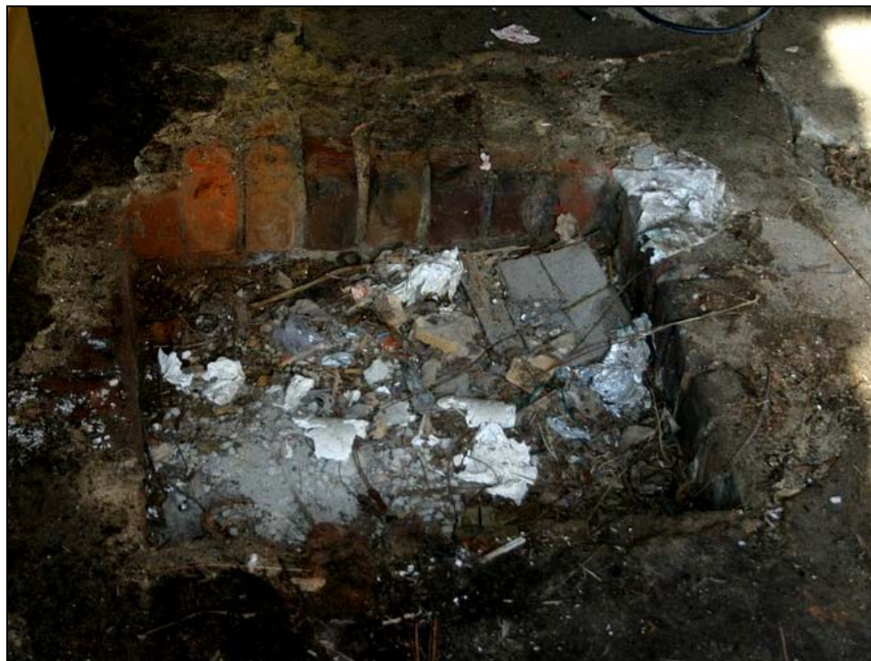
Figure 42: Fire pit, smokehouse. Penne Sandbeck, NCDOT, October 2010.
