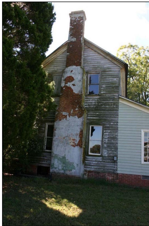
Figure 130: Smithwick-Green-Clark House, north elevation, original chimney. Penne Sandbeck, NCDOT, October 2010.
