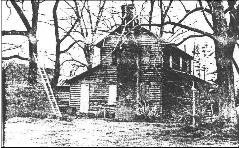
Figure 124: Hadley House, north elevation. Clifton Ellis for NCDOT, 2000.
