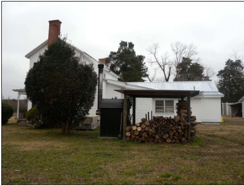
Figure 58: Roscoe Churchill Gorham House, woodshed and features of opposite side elevation. Brandon McCuin, Gray and Pape, February 2010.
