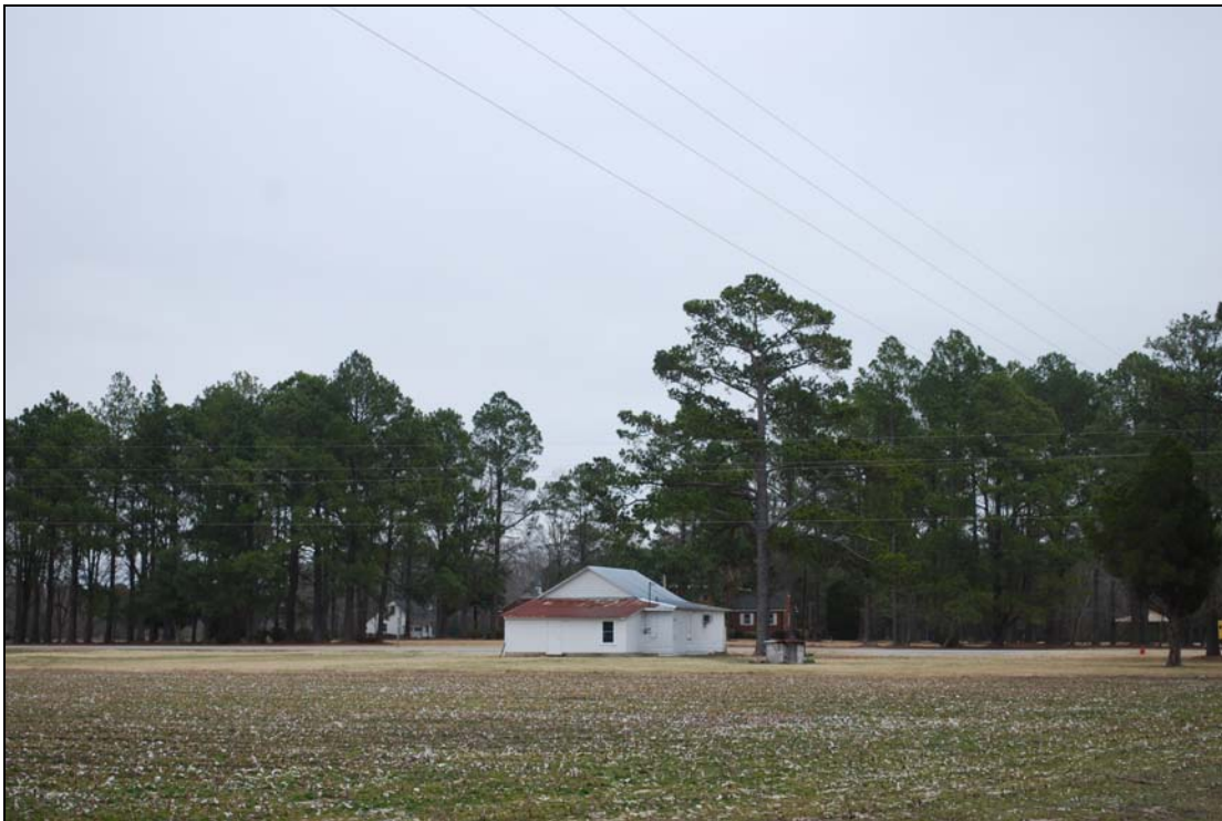
Figure 97: Corey's Store, west elevation. Kate Husband, NCDOT, February 2011.
