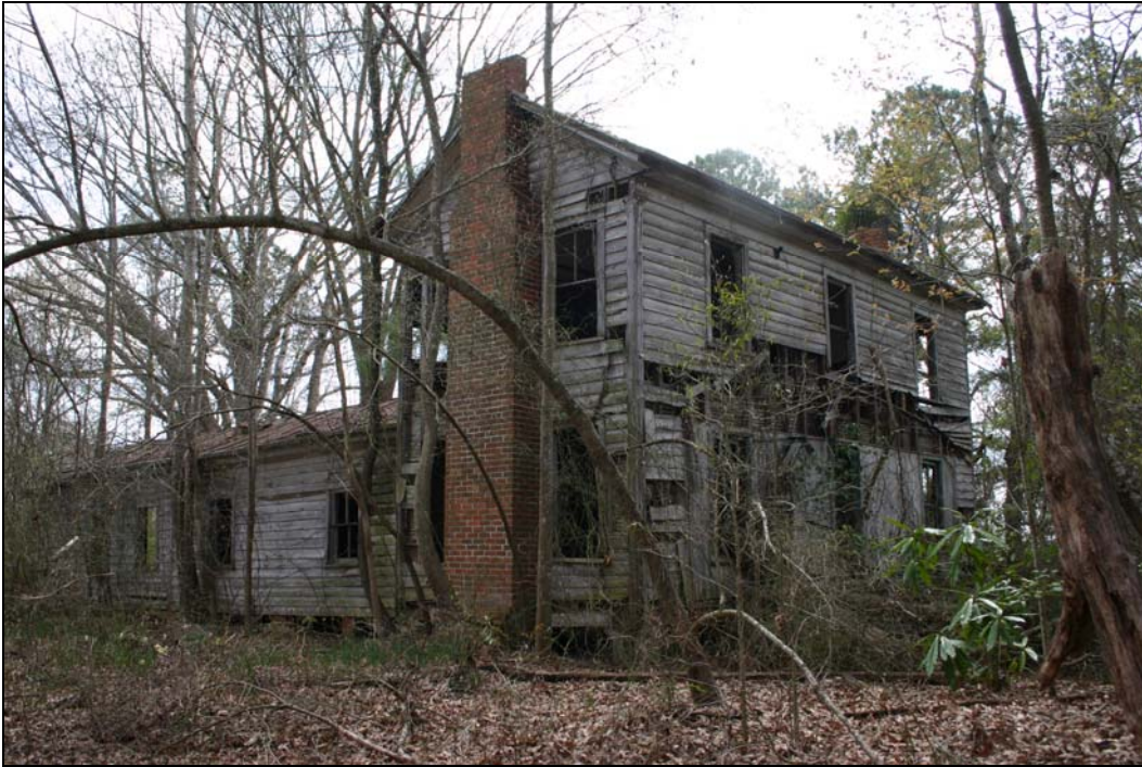
Property 5: No Address, North of North Roberson Road on US 17 PIN: 5679-55-6058 Loss of integrity and no architectural or archaeological significance.
