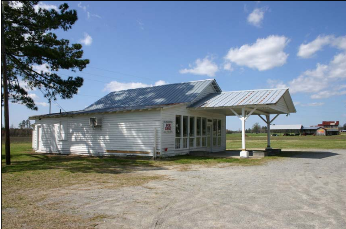
Figure 96: Corey's Store, east and south elevations. Penne Sandbeck, NCDOT, March 2010.
