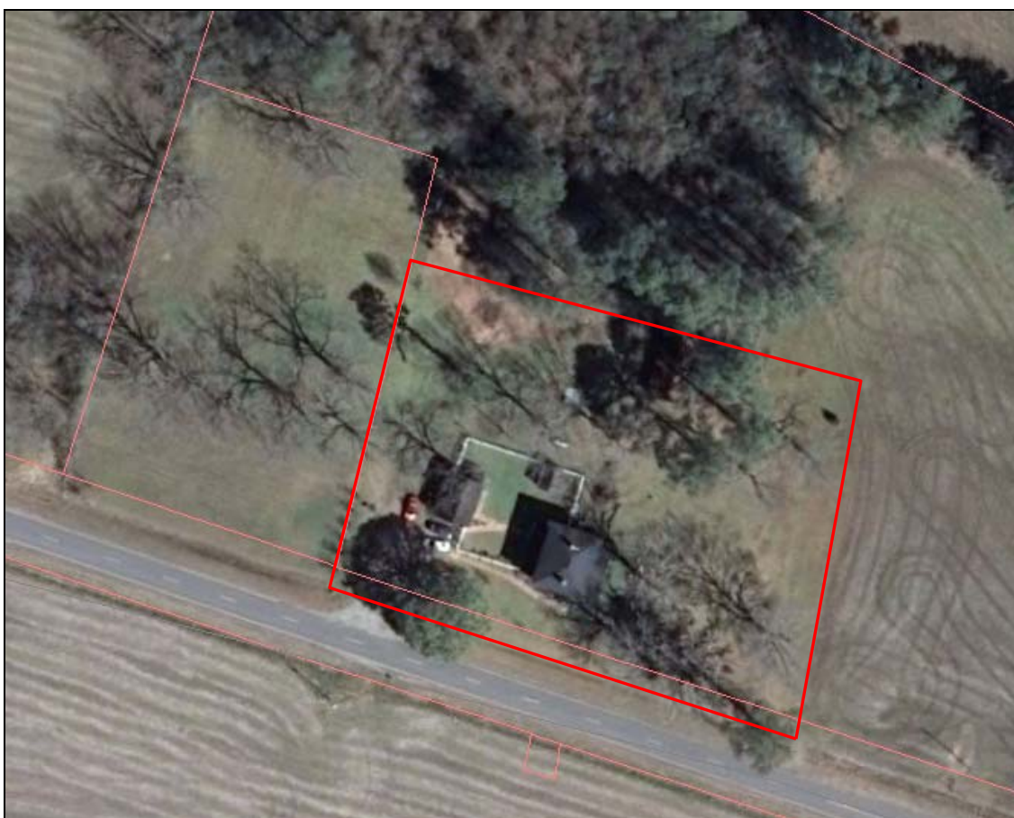
Figure 52: Proposed National Register Boundary, Thad Hodges House. Beaufort County GIS Tax Parcel Information
