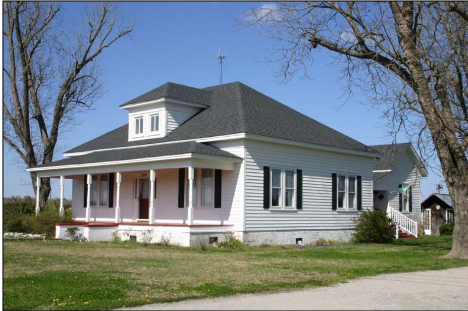
Figure 75: Benjamin Ward House, front and south elevations. Penne Sandbeck, NCDOT, March 2010.
