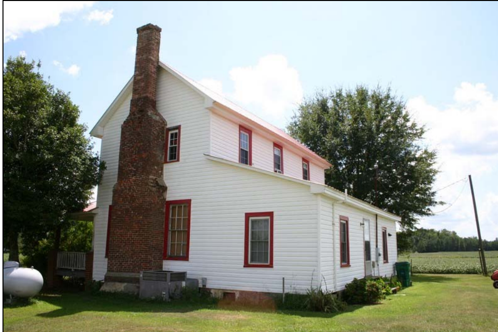
Figure 143: Woolard Perry House, north and west elevations. Penne Sandbeck, NCDOT, August 2010.
