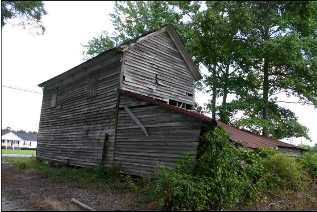
Figure 110: Holliday Store, south and east elevations. Penne Sandbeck, NCDOT, August 2010.
