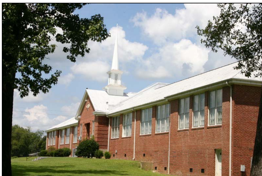
Figure 9: Former Old Ford School (now Old Ford Church of Christ), NC 171 at US 17 Junction. Penne Sandbeck, NCDOT, August 2010.
