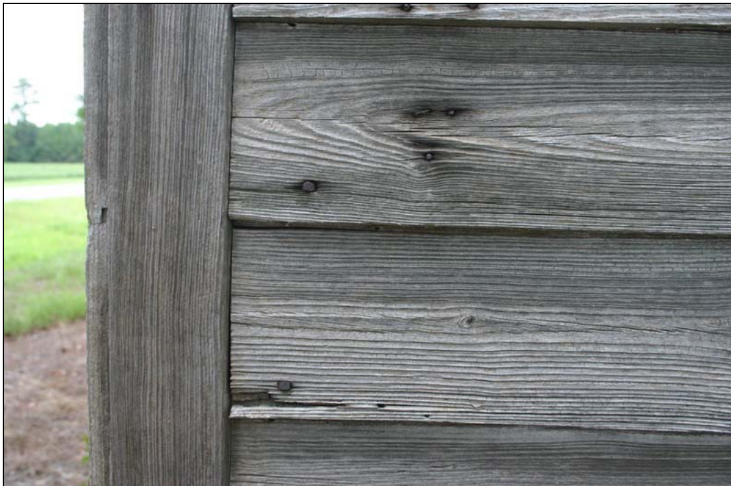
Figure 111: Holliday Store, sample of cut nail fasteners. Penne Sandbeck, NCDOT, August 2010.
