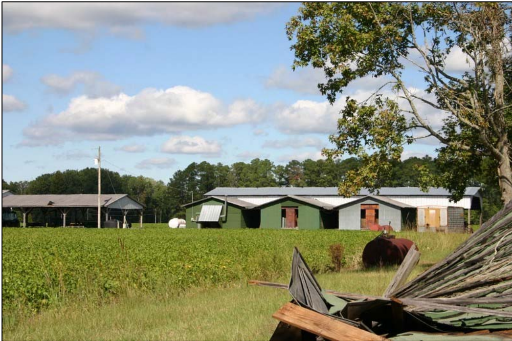
Figure 70: Bulk barns and open equipment sheds, looking northwest. Penne Sandbeck, NCDOT, August 2010.
