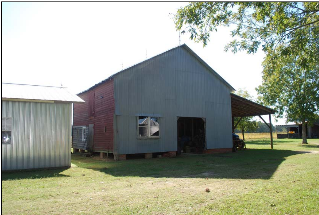
Figure 91: Livestock barn. Penne Sandbeck, NCDOT, October 2010
