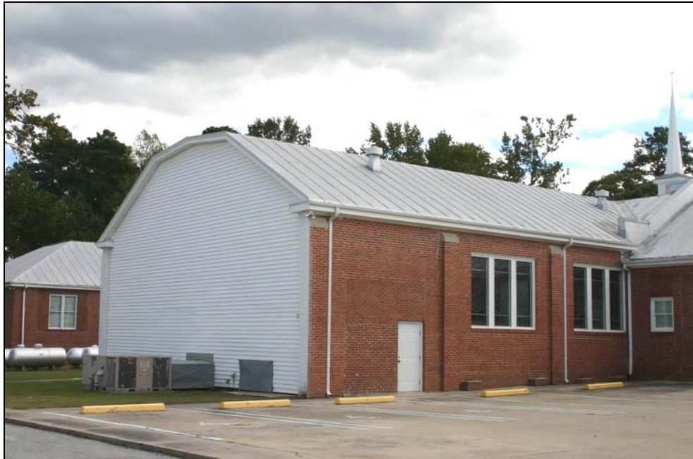
Figure 27: Auditorium wing, Old Ford School. Penne Sandbeck, NCDOT, October 2010.
