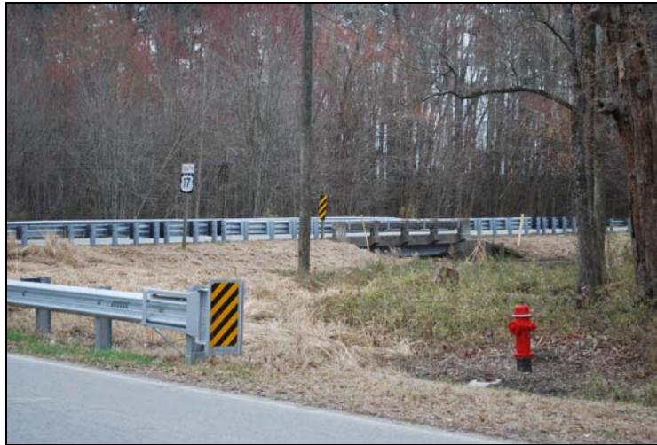
Figure 148: Bridge No. 56, Beaufort County. Kate Husband, NCDOT, February 2011.
