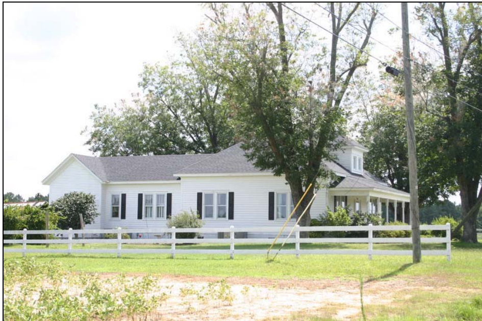
Figure 76: Benjamin Ward House, north elevation. Penne Sandbeck, NCDOT, August 2010.
