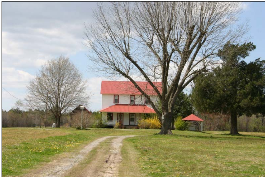
Figure 139: Woolard-Perry House, east façade. Penne Sandbeck, NCDOT, March 2010.
