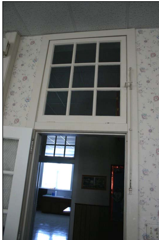
Figure 20: Example of hinged transom, Old Ford School. Penne Sandbeck, NCDOT, October 2010.
