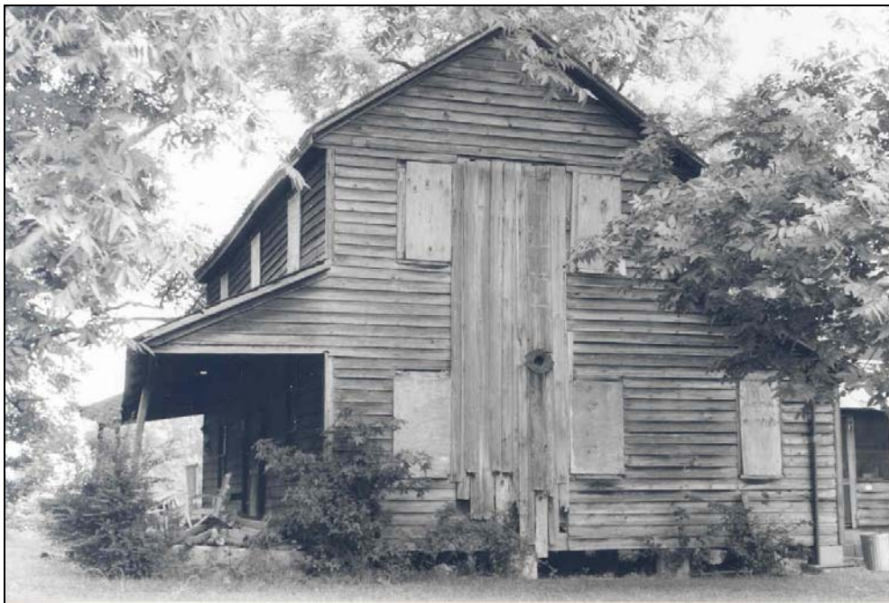
Figure 123: Hadley House, south elevation. Heather Fearnbach, NCDOT, 2001.
