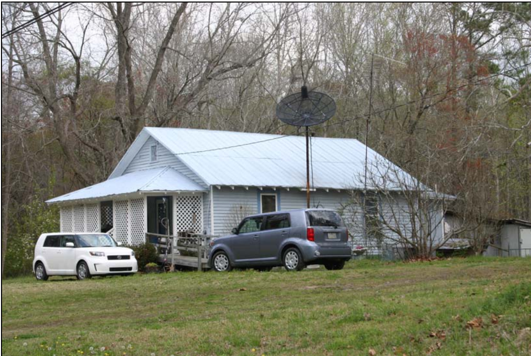
Property 6: 6498 US 17 PIN: 5679-44-5293 Common building type, no architectural or archaeological significance.
