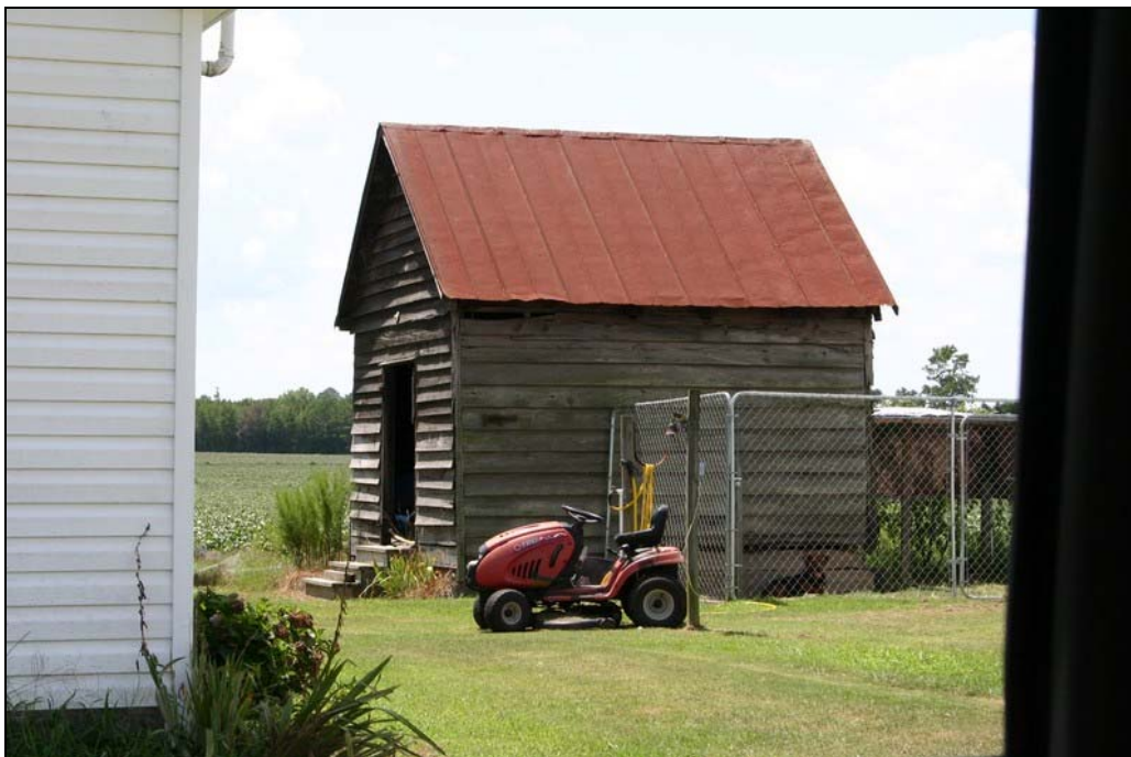
Figure 146: Woolard-Perry House, smokehouse. Penne Sandbeck, NCDOT, August 2010.
