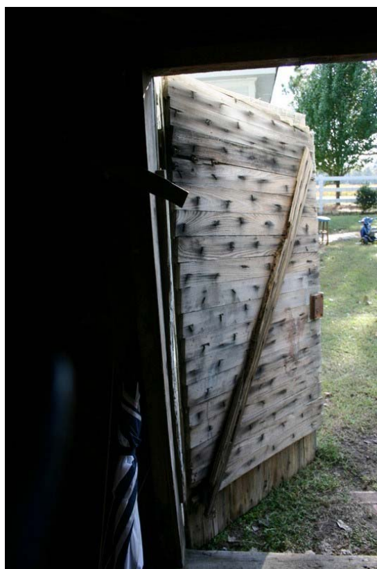
Figure 44: Smokehouse door. Penne Sandbeck, NCDOT, October 2010.
