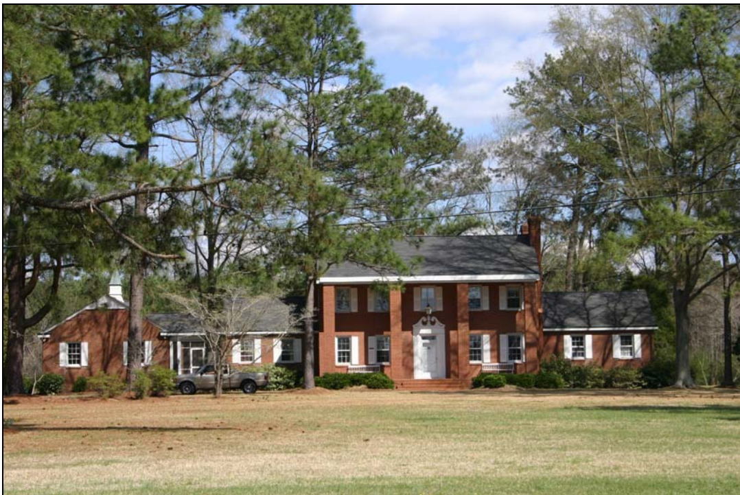
Figure 105: Lucien Peel House, east façade. Penne Sandbeck, NCDOT, March 2010.
