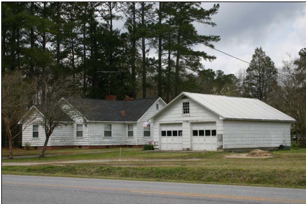
Figure 68: Oscar C. Hodges House, south and east elevations. Penne Sandbeck, NCDOT, August 2010.
