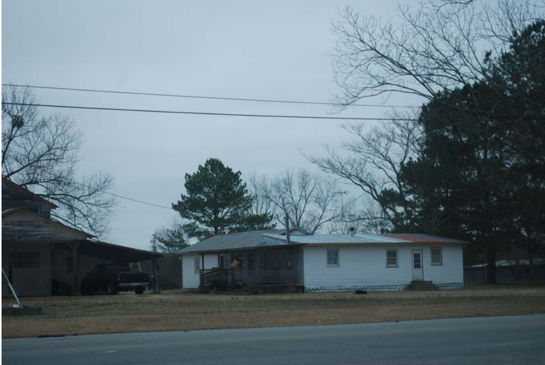
Figure 100: Mobile home connected to one-story house south of Rogerson's Store. Kate Husband, NCDOT, February 2011.
